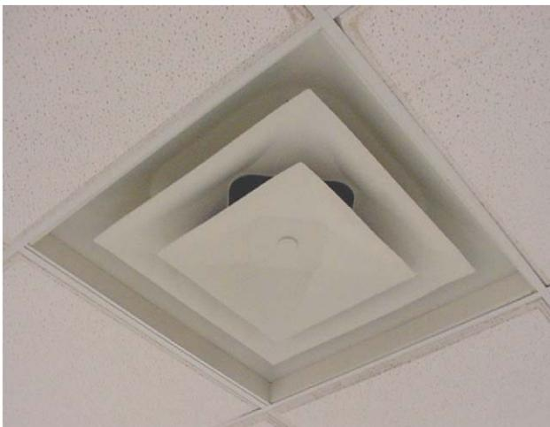
Fig. 3. Geometry of square cone diffuser.
